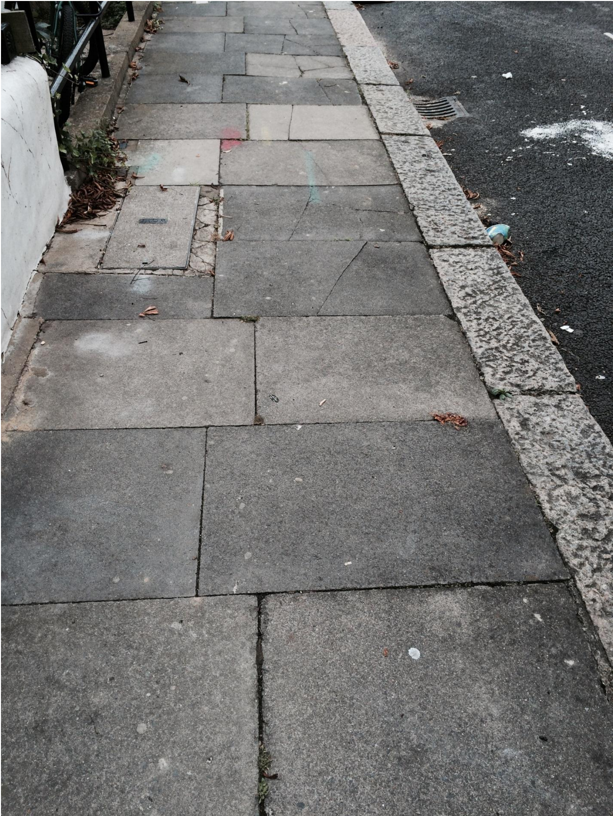
Case Study - A typical footway identified for repaving.
